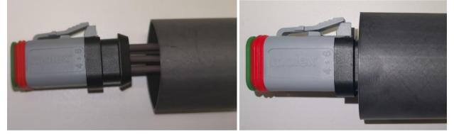
3. Apply heat and allow the heatshrink tubing to shrink around the housing and cables.
